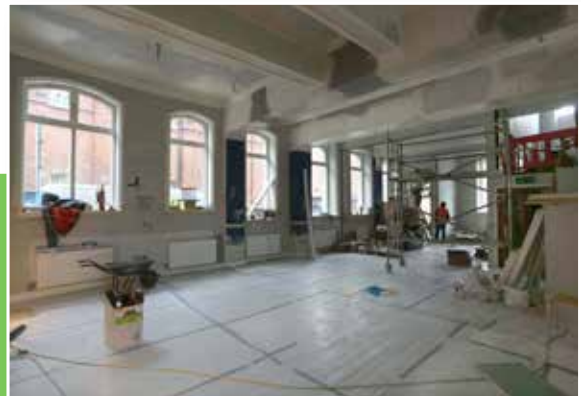
New FLAC office under renovation
